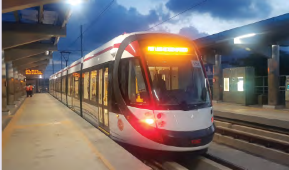
Figure 32.2: The Metro Express in Mauritius: this big infrastructure project is being completed within budget
